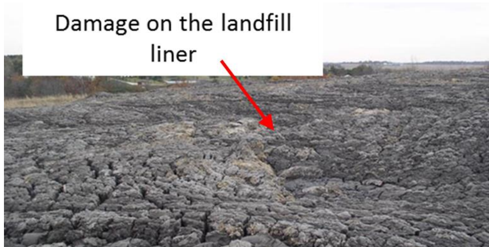
Figure 2.5 Desiccation cracks on mud used as landfill top cover at Pekin Landfill Illinois (Source: https://www.istc.illinois.edu/research/resource_recovery/mud_to_parks_il_river_project/photos/pekin_landfill/ )
