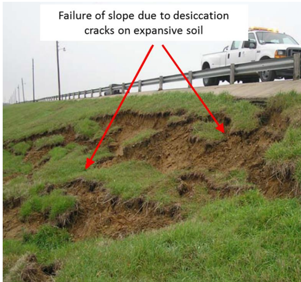
Figure 2.4 Slope failure triggered by desiccation cracks of expansive soils (After McCleskey et al. 2008)
