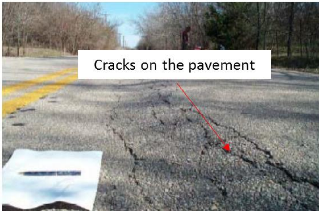
Figure 2.3 Pavement distress caused by swell shrink soil (After Puppala et al. 2011)
