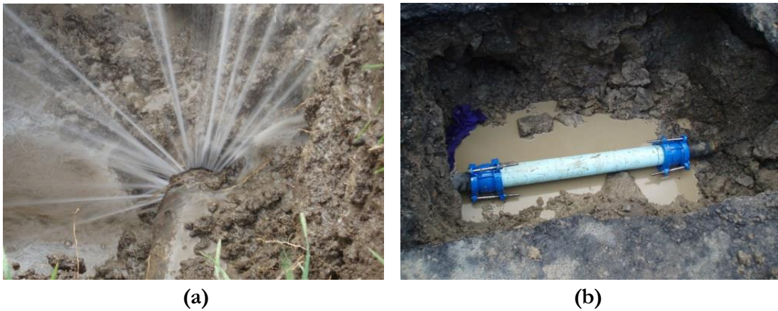
Figure 3-2 Failure of water pipe: (a) Exposed circumferential fractured pipe; (b) Pipe replacement with PVC section
