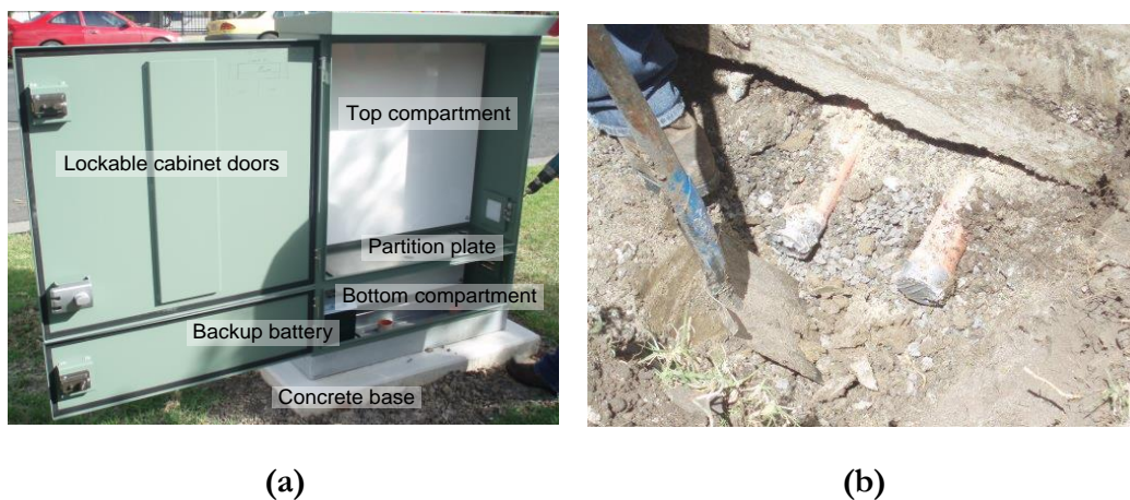
Figure 3-25 Metal cabinet at Altona North: (a) layout of the cabinet; (b) conduit bends at the base of the cabinet
