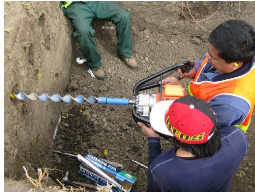
Figure 3-53 Horizontal drilling in preparation of sensor installation
