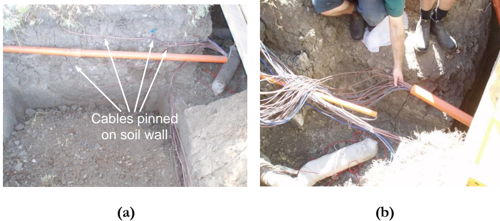
Figure 3-40 Wiring at Altona North: (a) sensors cables pinned to the wall; (b) sending of sensors cables through conduits
