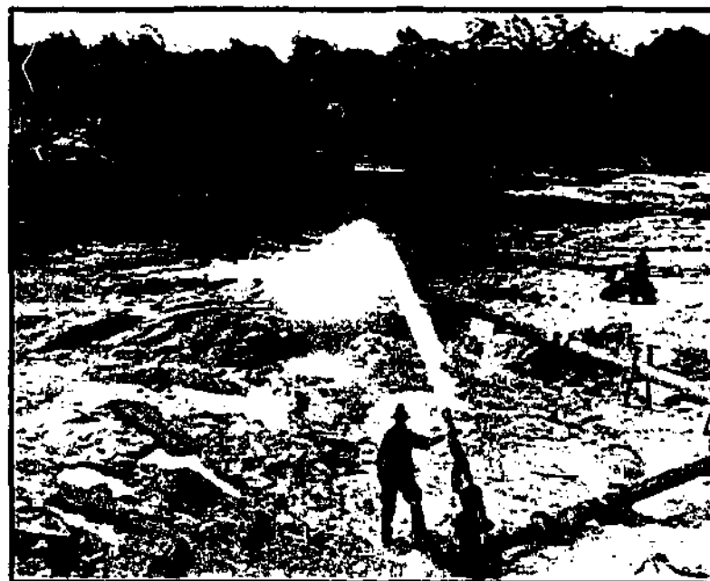
Plate 4.11: An example of the sluicing operations on the Ringarooma River (Source: St Helen's historic library)
