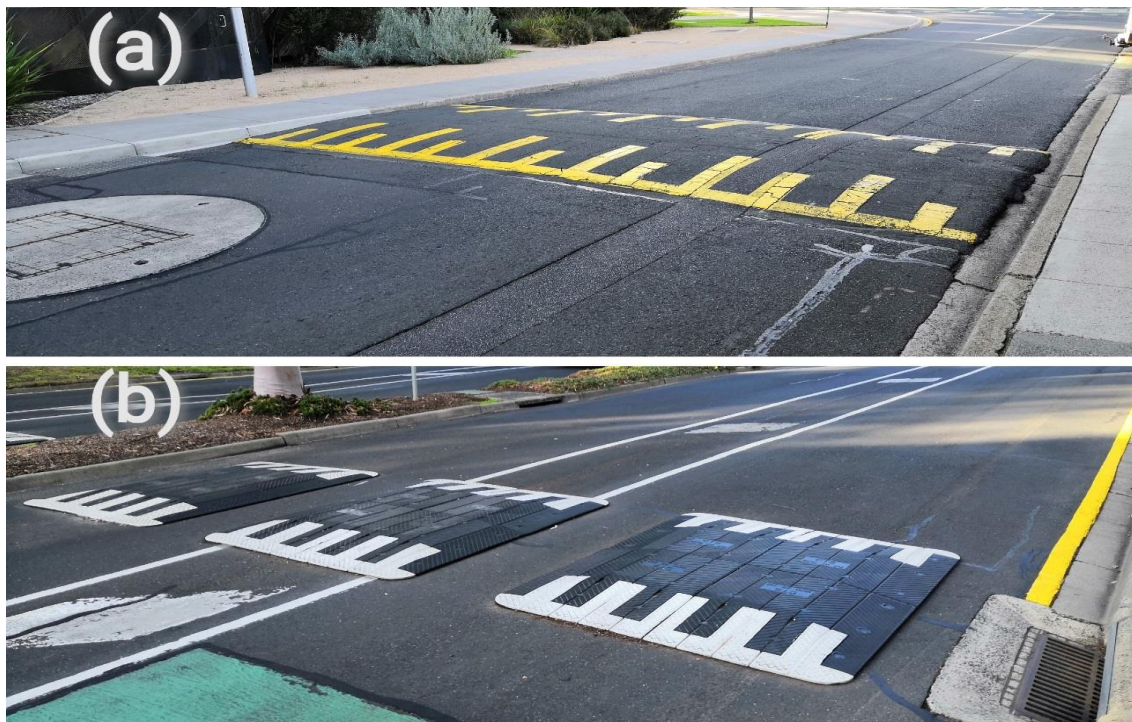
Figure 2-2: Common types of traffic calming measures at Monash University Clayton; (a) speed humps, (b) speed lumps/cushions
