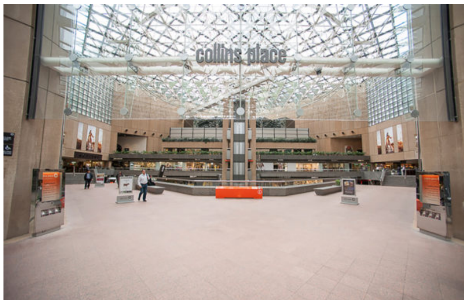
Figure 5. Entrance to Collins Place showing space-frame ceiling. Case Mealan, Collins Place, digital photograph, 2007, accessed October 25, 2016, http://xvkjc2tqpxzx5u5g3wwwmx5xz.wpengine.netdna-cdn.com/wp-content/uploads/2016/09/AMP-Collins-Place-35-Collins-St-2620V_1400x900_web8-600x386.jpg .
